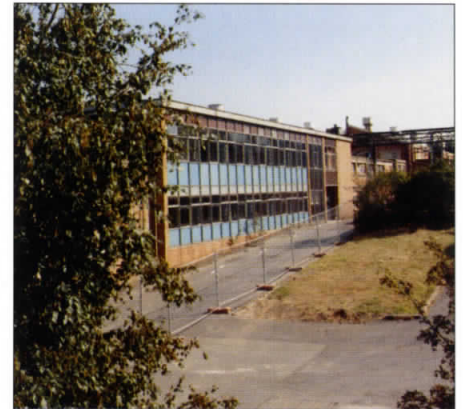
Tech Block and Stalag prior to demolition
