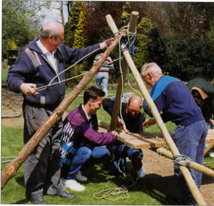
Bridge building in action!
