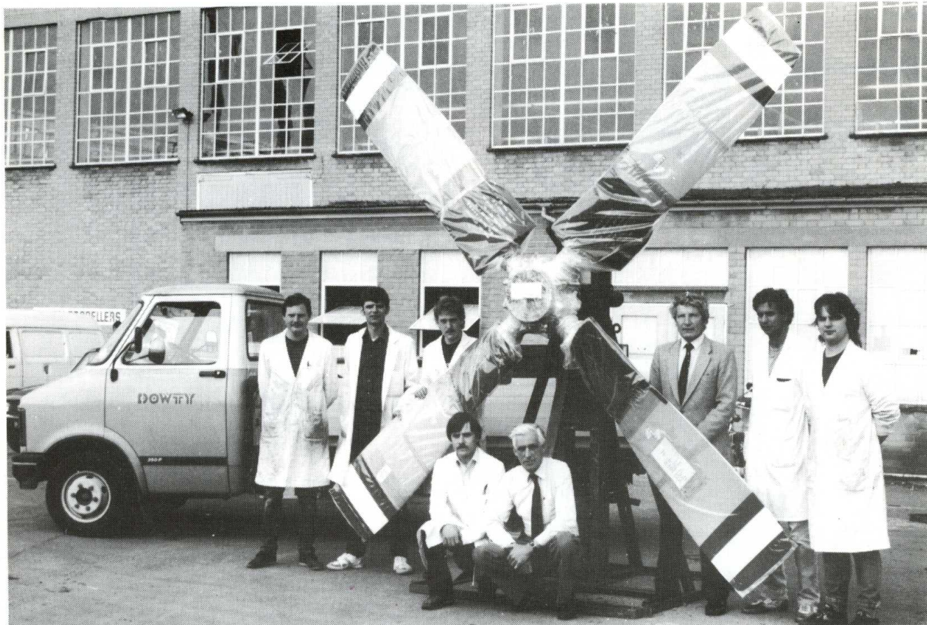
Despatch on 26 June of the first Lockheed C-130 Hercules propeller overhauled at Dowty RotoI
