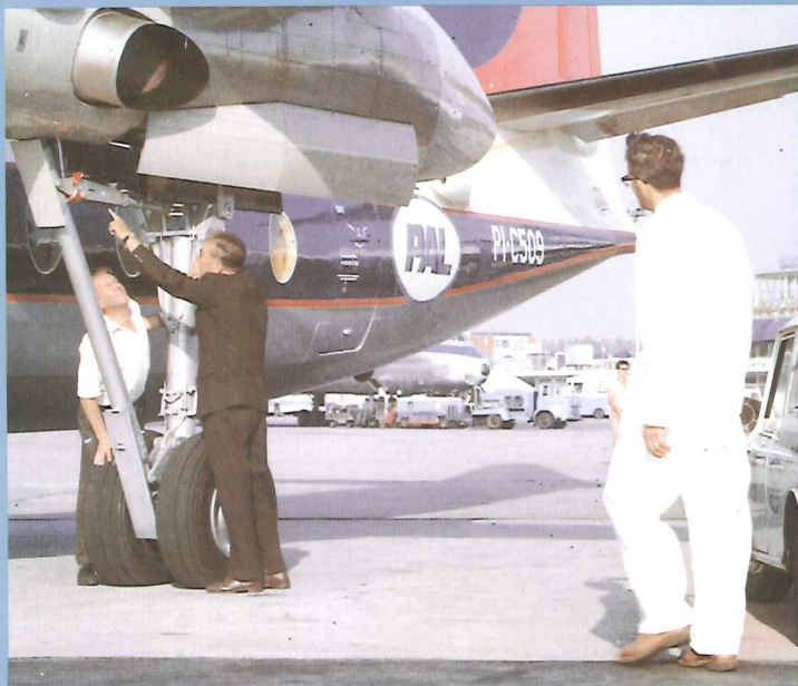
Field servicing of Fokker F27 main landing gear
